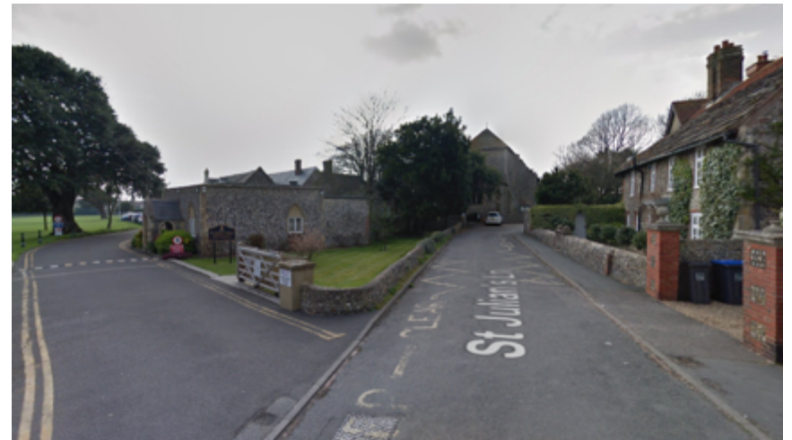
Fig 6: View towards church and rectory from St Julian's Lane
