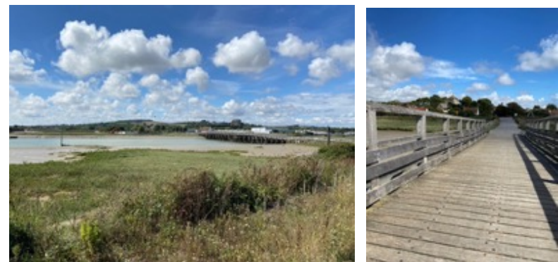
Fig 7: Old Shoreham Toll Bridge
