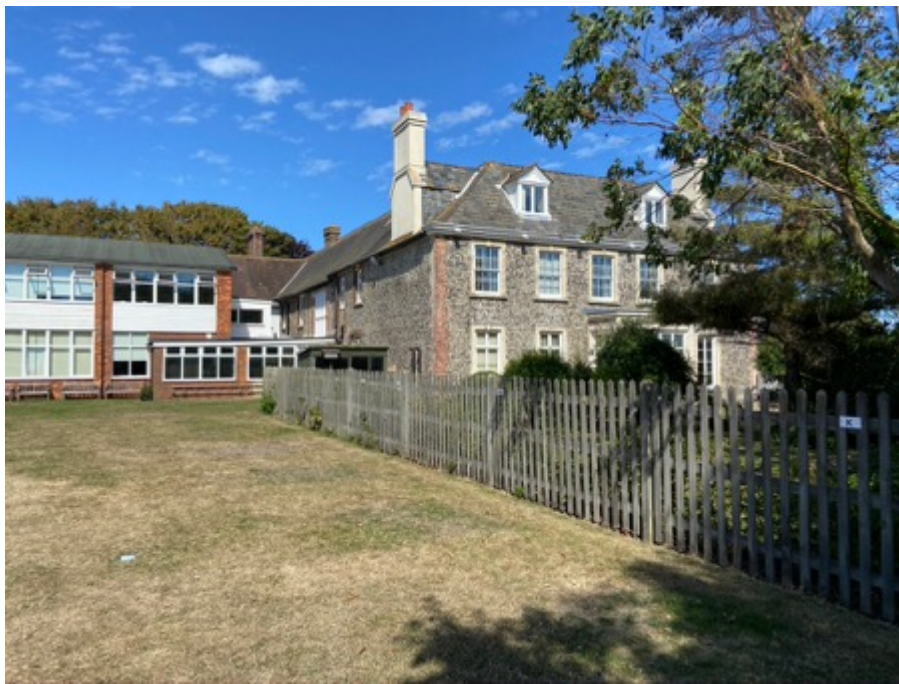
Fig 14: Knapped and coursed flint, slate roof
