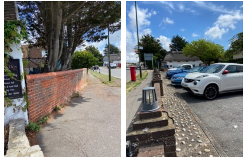
Fig 34: Modern inappropriate brick wall and boundary treatments
