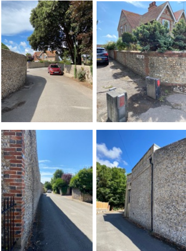
Fig 19: Historic flint walls
