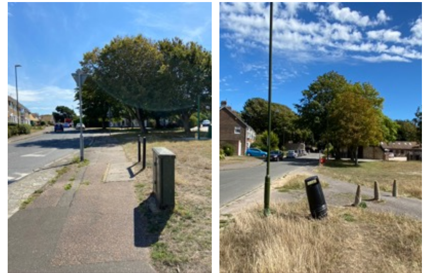
Fig 32: poor quality street furniture and surfaces along St Julian's Lane
