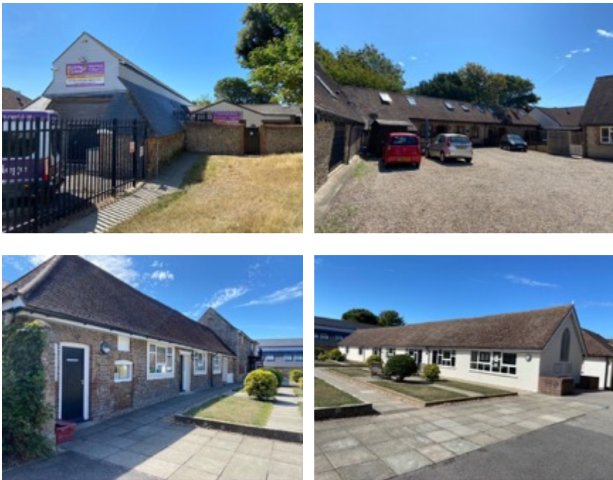
Fig 16: Former agricultural buildings west and northwest of Shoreham College
