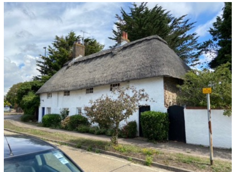
Fig 16: Thatch, render, brick and flint concealing earlier timber frame at Connaught Avenue
