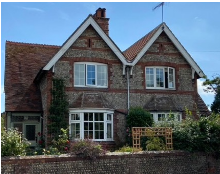
Fig 30: Modern uPVC windows to unlisted historic buildings
