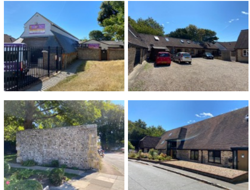
Fig 11: Former agricultural buildings associated with the manor house
