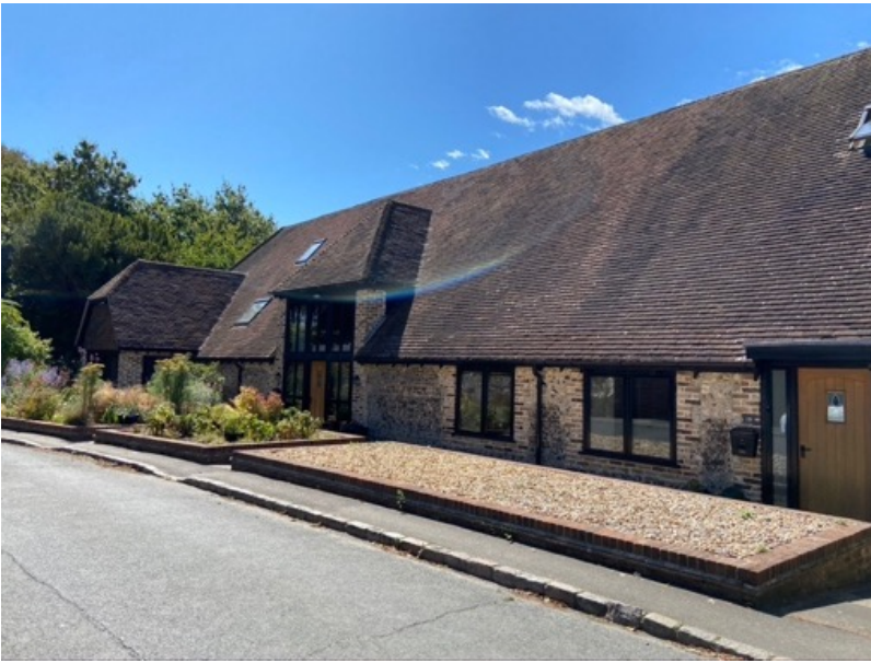
Fig 33: Domestic character of barn and setting
